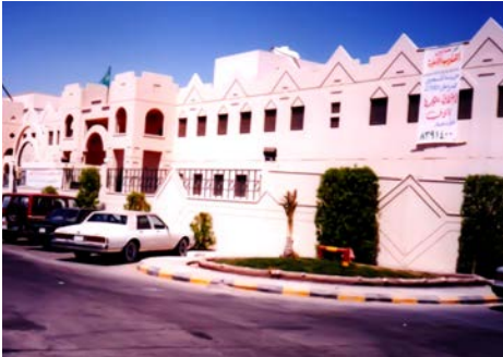
AL TATHEEB PRIVATE SCHOOL BUILDING
